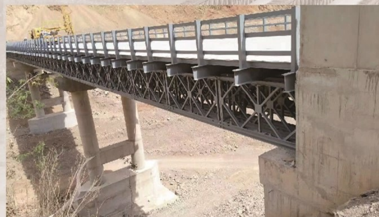
上承式贝雷桥 Deck Bridge
